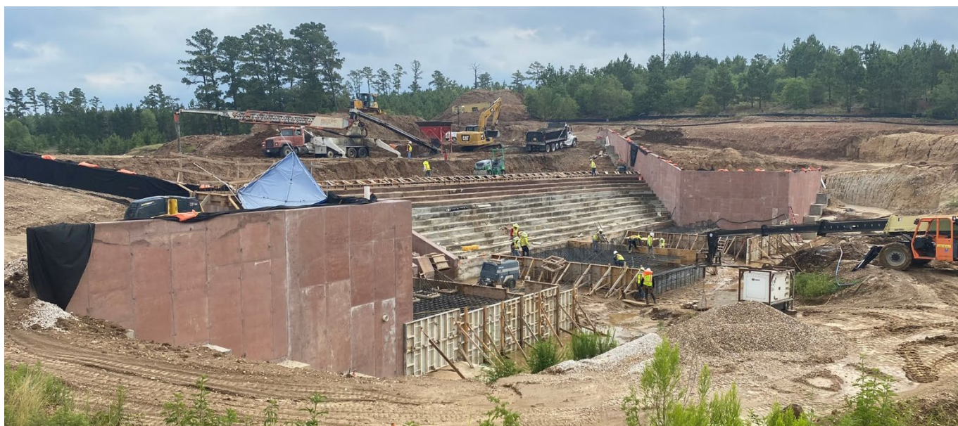
Reconstruction of the Bastrop State Park Dam
