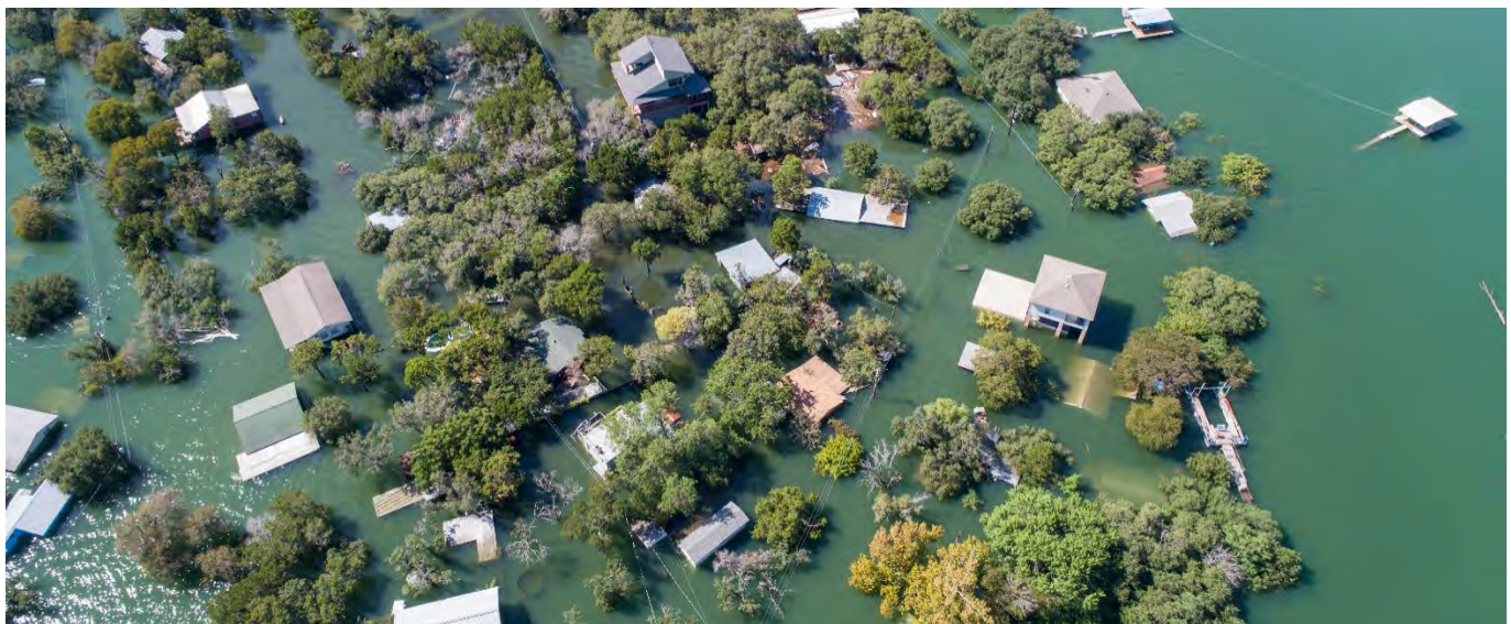
Impact to structures after flooding in the Central Texas Region. Source: Shutterstock
