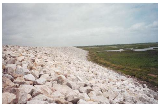
Example Coastal Protections – Sea Wall and Rock Riprap Revetment
