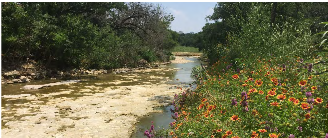
Example Channel Improvements - Shoal Creek Channel Improvement and Restoration Project, Austin
