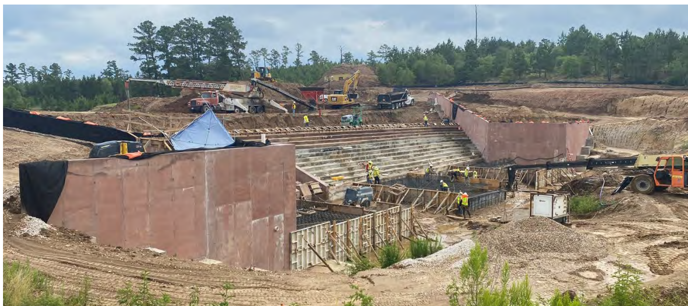
Reconstruction of the Bastrop State Park Dam
