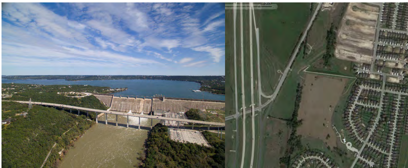
Example of Large Flood-Control Reservoir - Lake Travis, LCRA and Example of Regional Detention - Upper Brushy Creek WCID Flood Detention Structure No. 20
