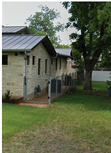
Figure 3: Example of Elevated Finished Floor
