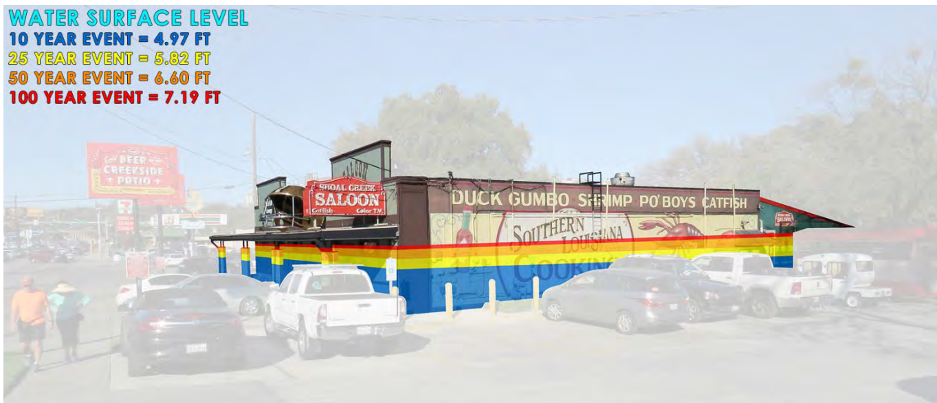
Source: City of Austin Lower Shoal Creek Risk Reduction Study – Flood Hazard Analysis of the Shoal Creek Saloon
