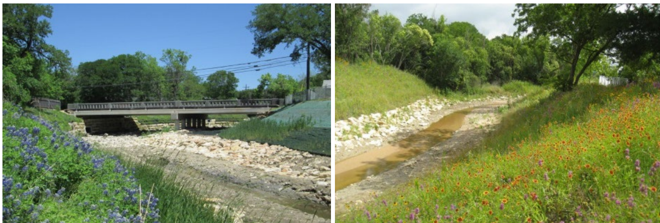
Example Channel and Bridge Upgrade Project with Natural Channel Design Elements, Fort Branch Creek, Austin
