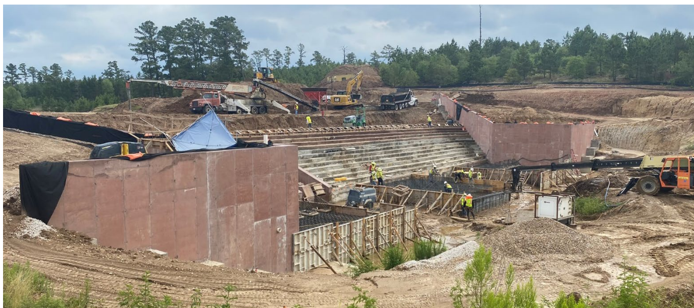
Reconstruction of the Bastrop State Park Dam
