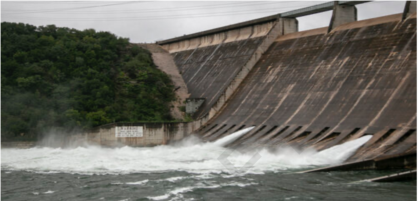
Source: Lower Colorado River Authority Mansfield Dam flood gates
