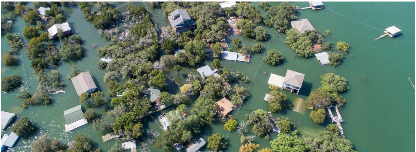
Impact to structures after flooding in the Central Texas region. Source: Shutterstock.
