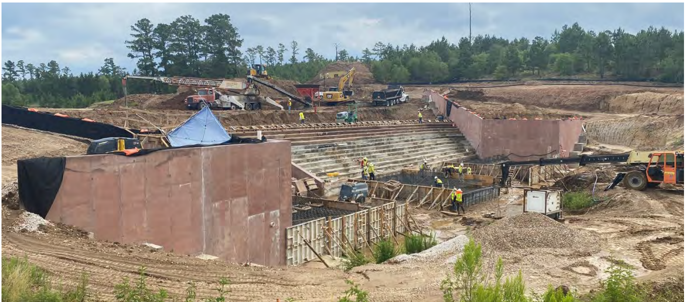
Reconstruction of the Bastrop State Park Dam
