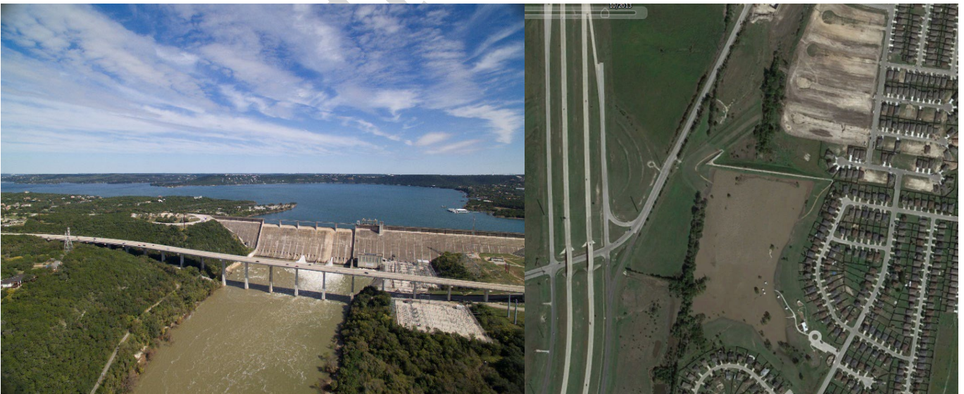
Example of Large Flood-Control Reservoir - Lake Travis, LCRA and Example Regional Detention - Upper Brushy Creek WCID Flood Detention Structure No. 20
