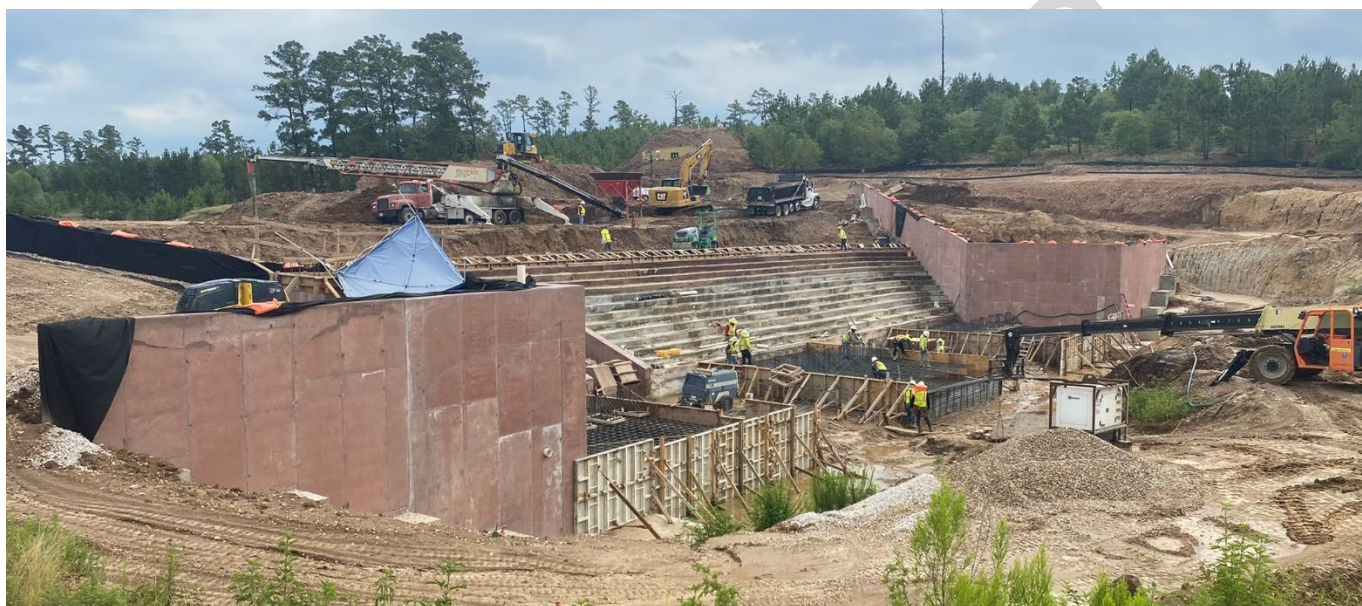
Reconstruction of the Bastrop State Park Dam
