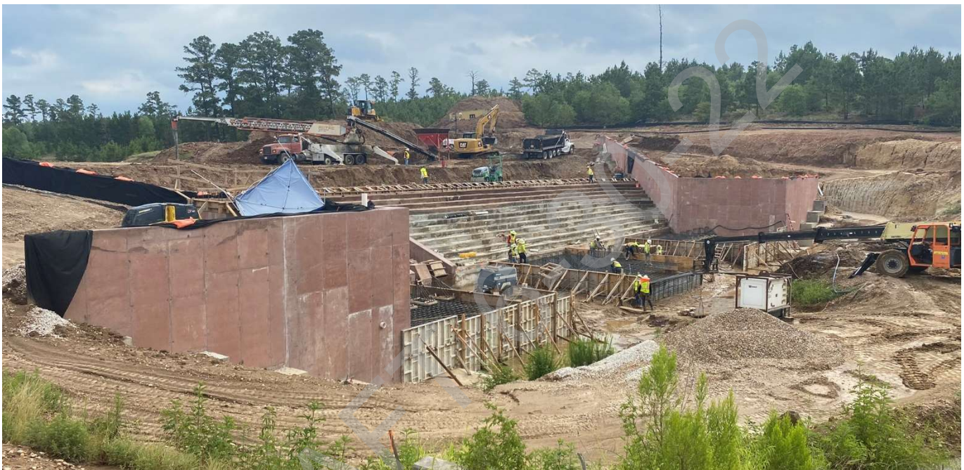
Reconstruction of the Bastrop State Park Dam
