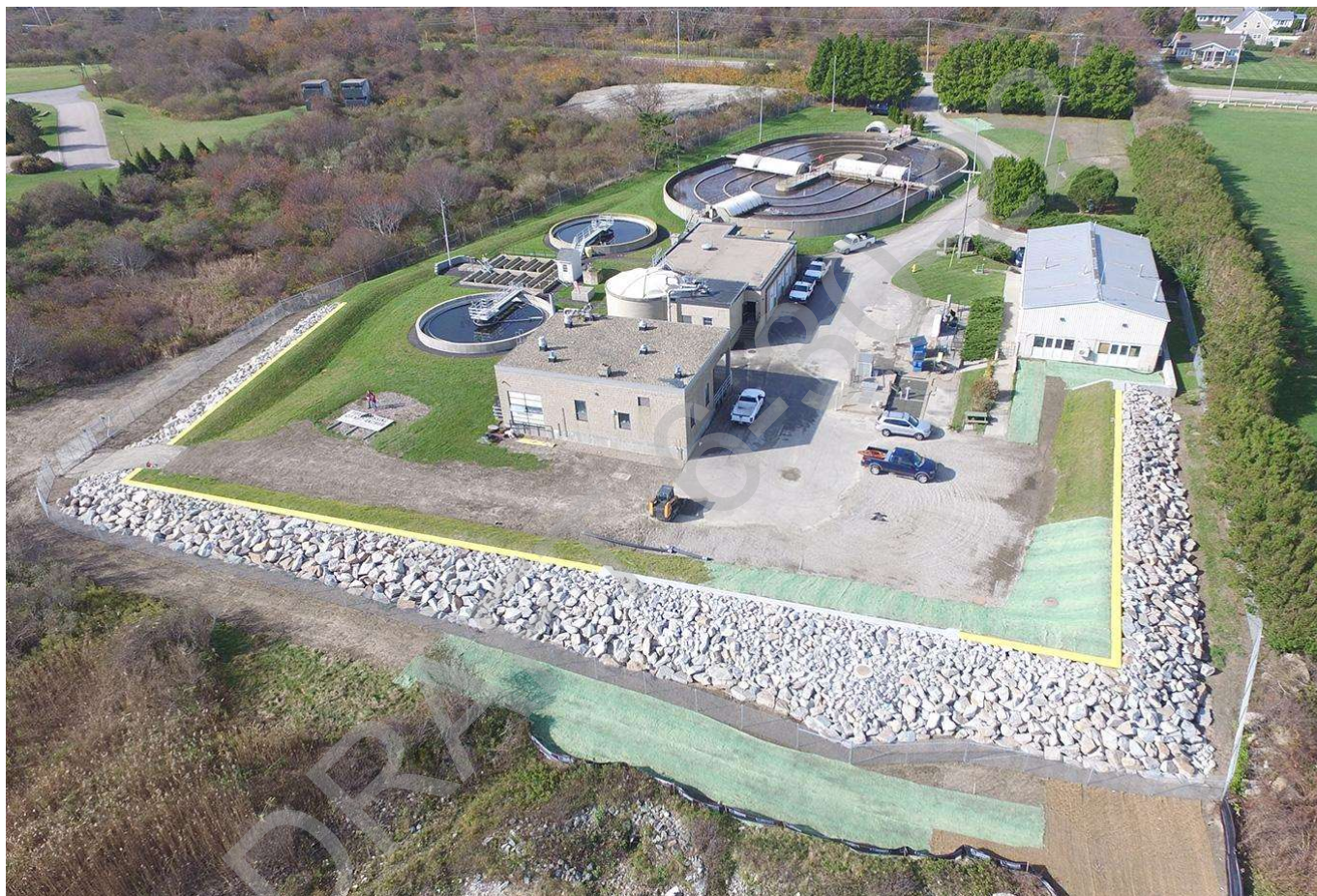
Example: Wastewater Treatment Facility Floodproofing (Source: RT Group, Inc.)
