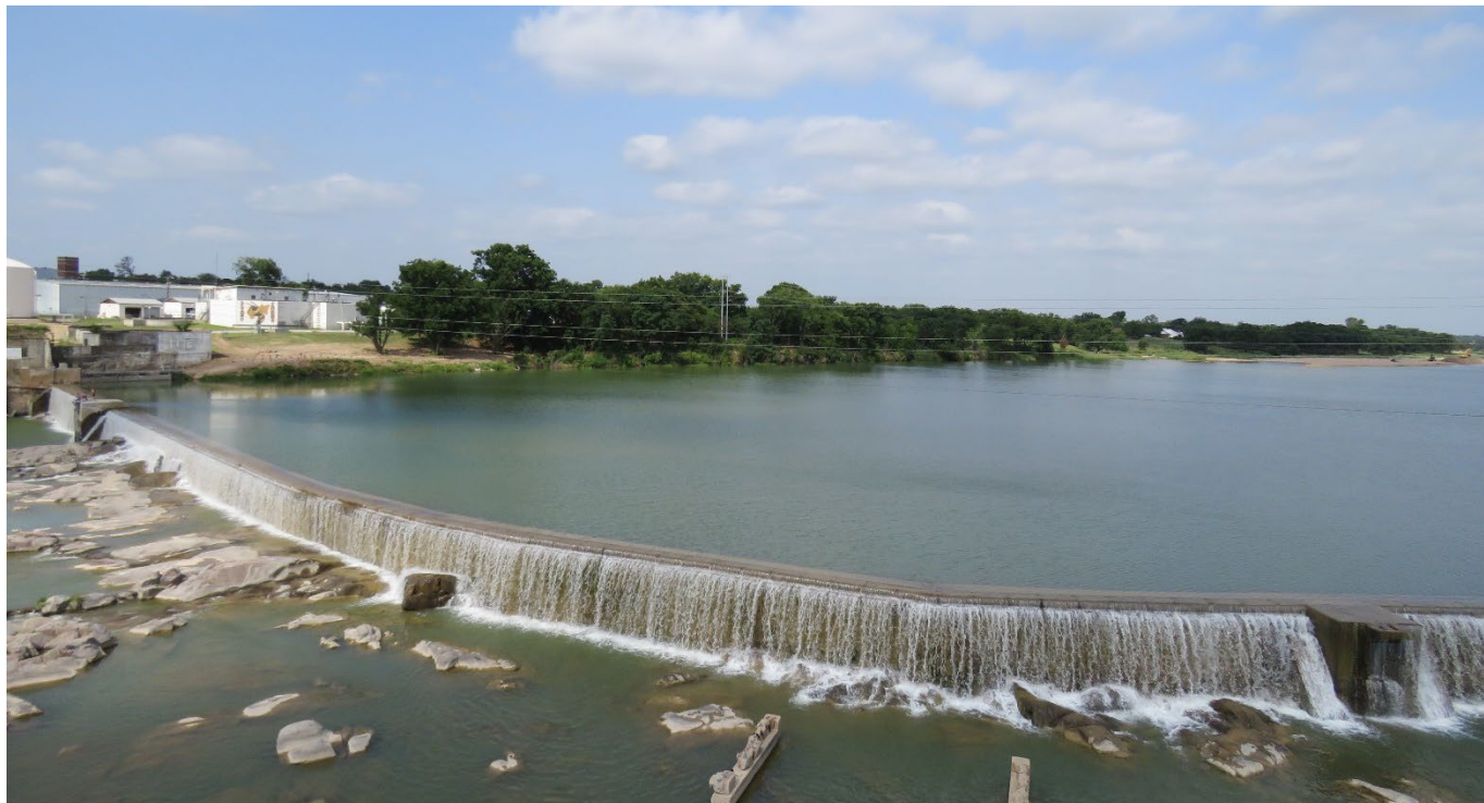
Source: Llano River Dam, Llano, TX
