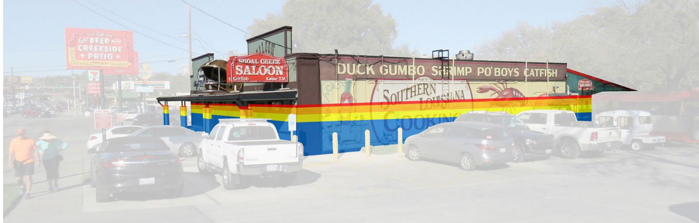
Source: City of Austin Lower Shoal Creek Risk Reduction Study – Flood Hazard Analysis of the Shoal Creek Saloon
