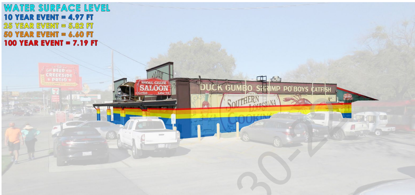
Source: City of Austin Lower Shoal Creek Risk Reduction Study – Flood Hazard Analysis of the Shoal Creek Saloon
