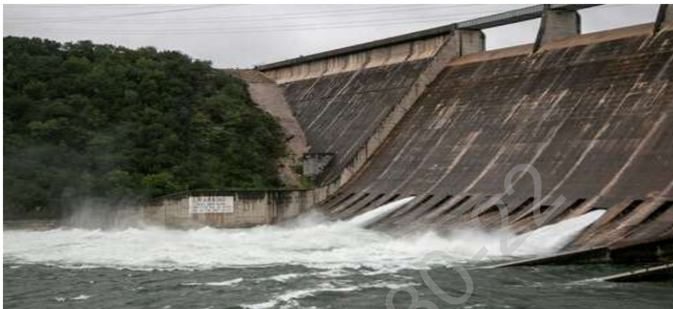
Source: Lower Colorado River Authority Mansfield Dam Flood Gates
