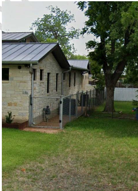
Figure 3: Example of Elevated Finished Floor
